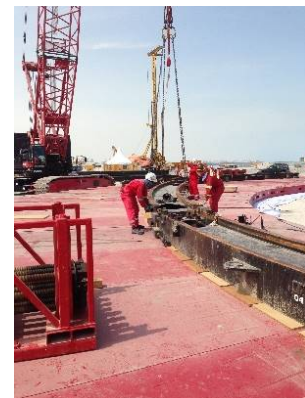
Photos 3 & 4: Outer ring complete and bolts torqued 12/08/14, Bracing installed to tie two rings together
