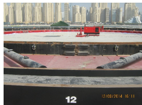
Photos 3 & 4: Outer ring complete and bolts torqued 12/08/14, Bracing installed to tie two rings together
