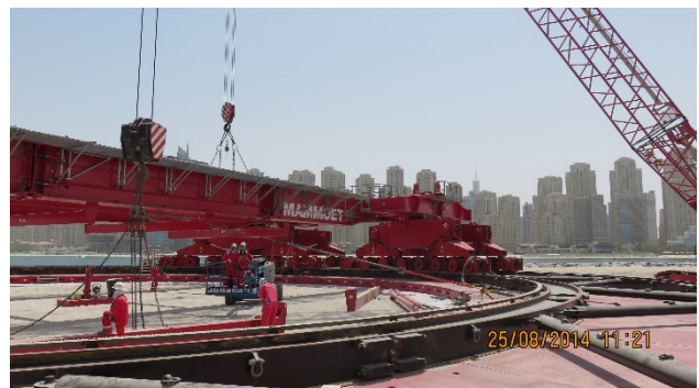
Photo 3: installing winch beams between front and rear.
