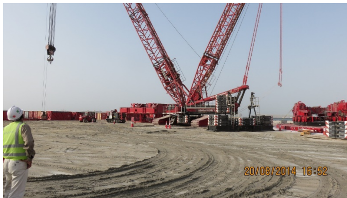
Photo 2: counterweight support frame and front sections installed 23/08/14
