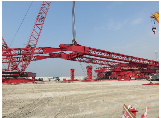
Backmast and support legs in place. 070914
