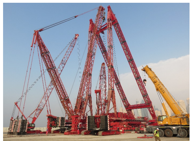
Backmast and support legs in place. 070914
