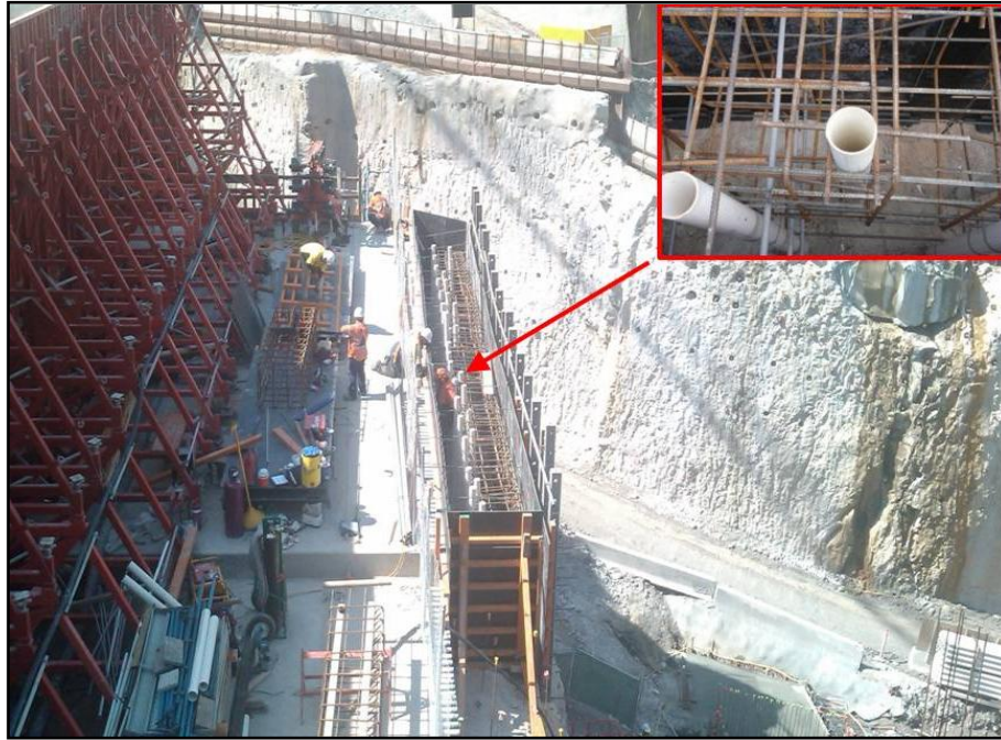
Figure 6: Collar pipes and reinforcement.
