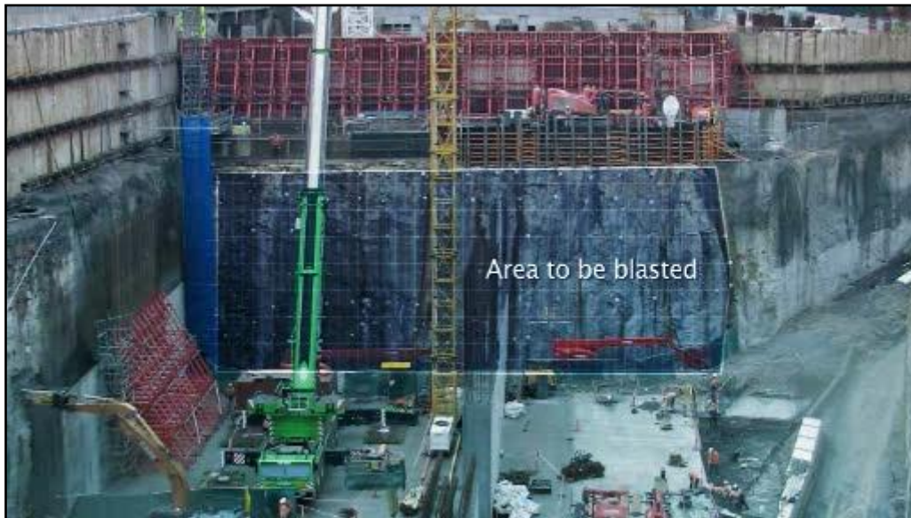
Figure 3: Rock Wedge to be removed.
