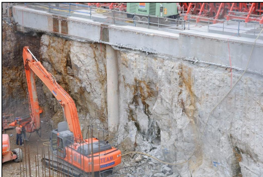
Figure 10: Embedded concrete piles remain intact.
