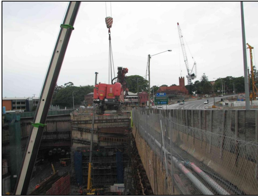
Figure 7: Lifting in the drill rig.
