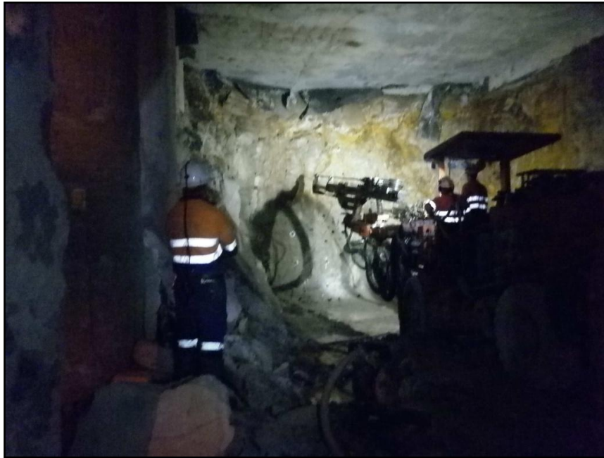
Figure 11: Drilling of the first breakthrough blast.
