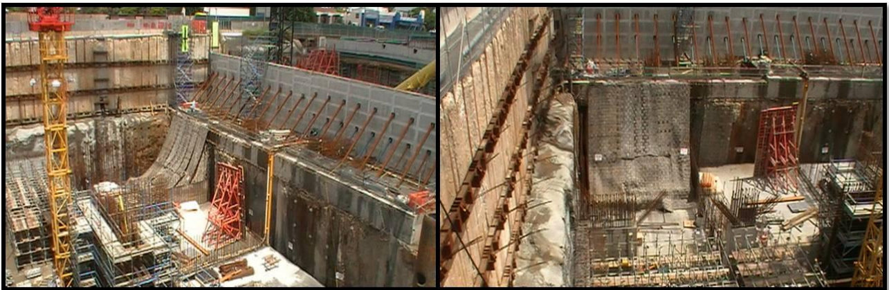
Figure 12: Blast mats in place for the first breakthrough.
