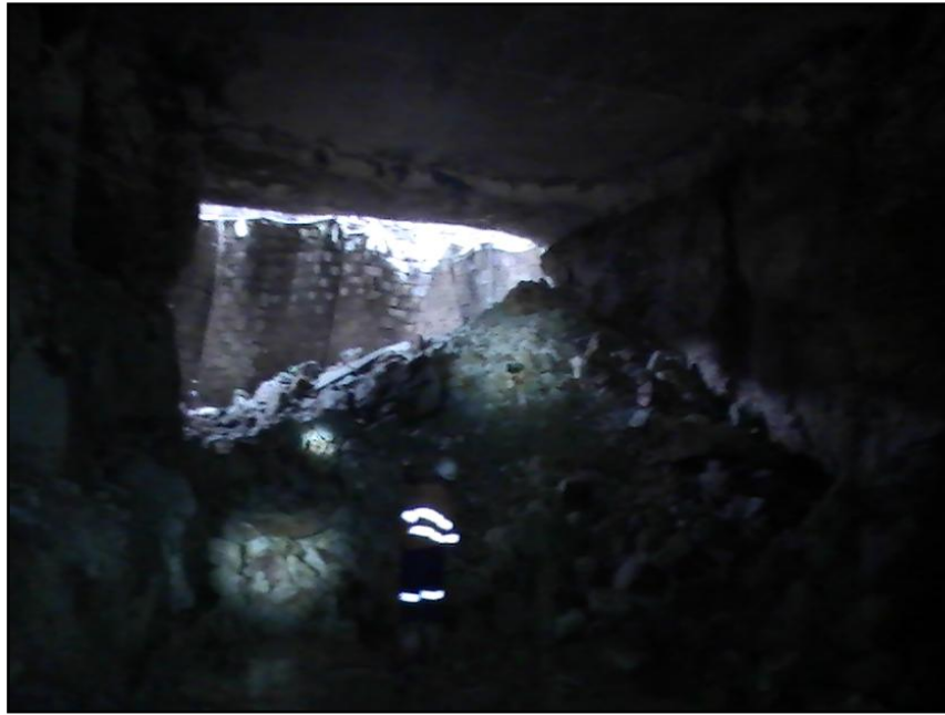
Figure 13: Inspecting the blast, a successful breakthrough.
