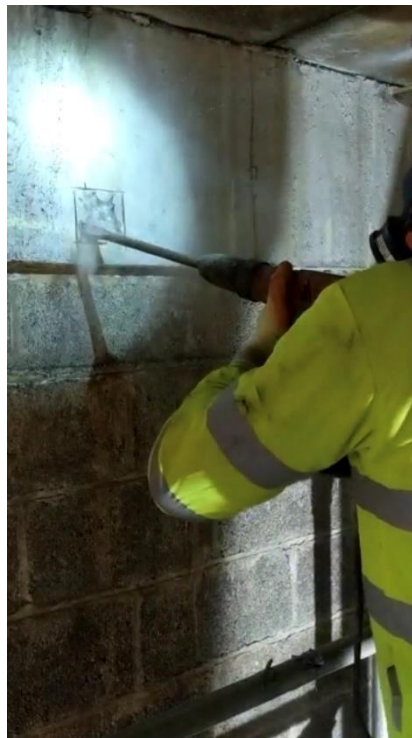
Chiselling to expose re-bar
