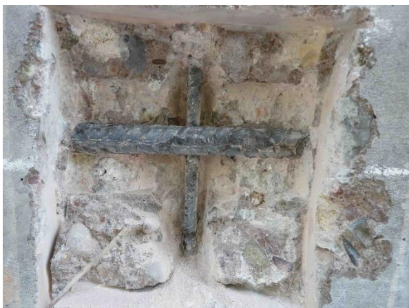
Exposure of reinforcement
